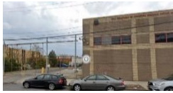
Garage Roof and HVAC Upgrade
