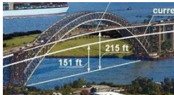
Raising Bayonne Bridge
