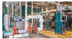
Boiler Upgrade at O'Dwyer Gardens
