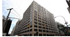
201 Varick Federal Building Tenant Backfill
