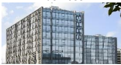
Intel Campus Sarjapur Ring Road Building 3
