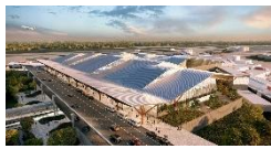
Pittsburgh International Airport (TMP)
